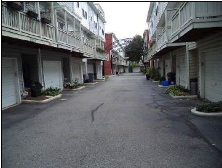
Photo #2: Additional asphalt maintenance repairs
