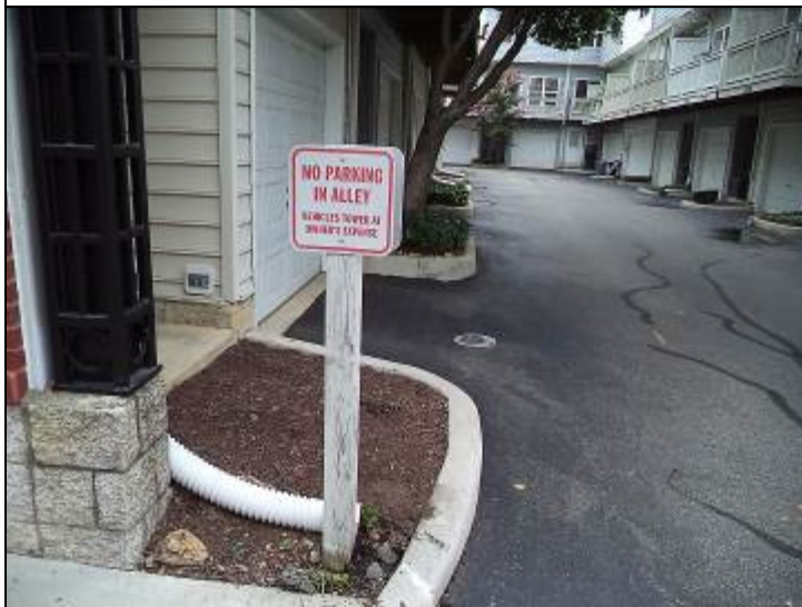
Photo #3: Consideration should be given to re-painting the posts.
